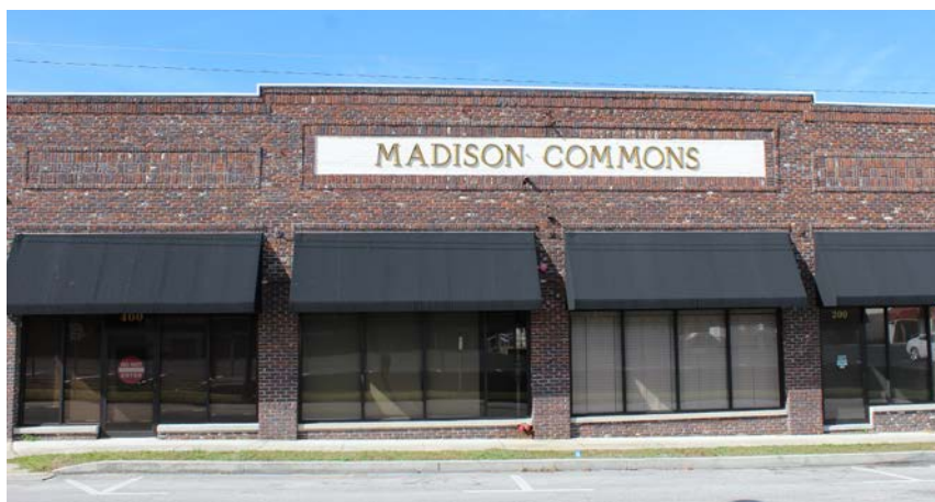
Madison Commons is a successful example of an adaptive reuse project, transitioning from a millwork to innovative office and commercial space
